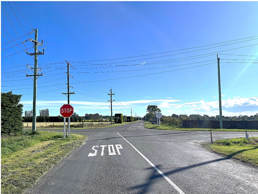
Figure 3: Rural crossroad in New Zealand with oversize Stop signs.
